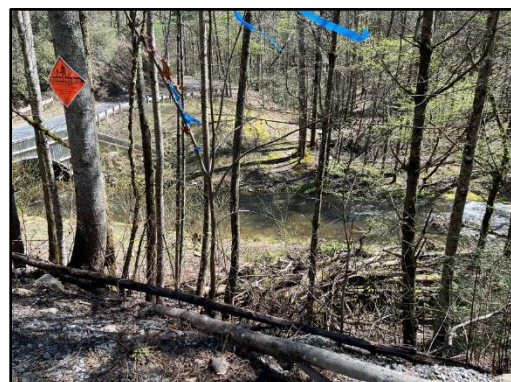
Figure 6 shows the culvert on the left side of the image, with the creek to the left as the holding line.
